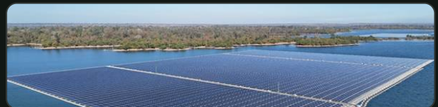
9.16 MW DC Mega Plant BTM BHIWANI, HARYANA
