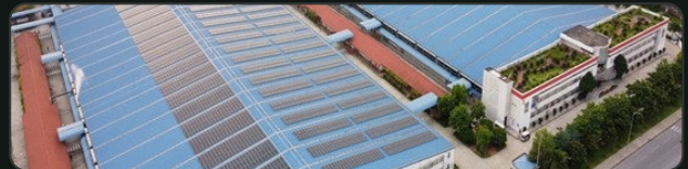
2.5 MW Desert Solar Project HEMRA, BIKANER, RJ
