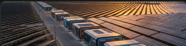
2.5 MW DC / 2 MW AC Ground Solar HANUMANGARH, RJ
